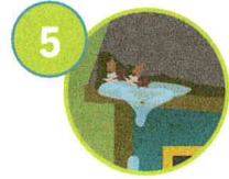
5 Clogged rain gutter (home and street)
